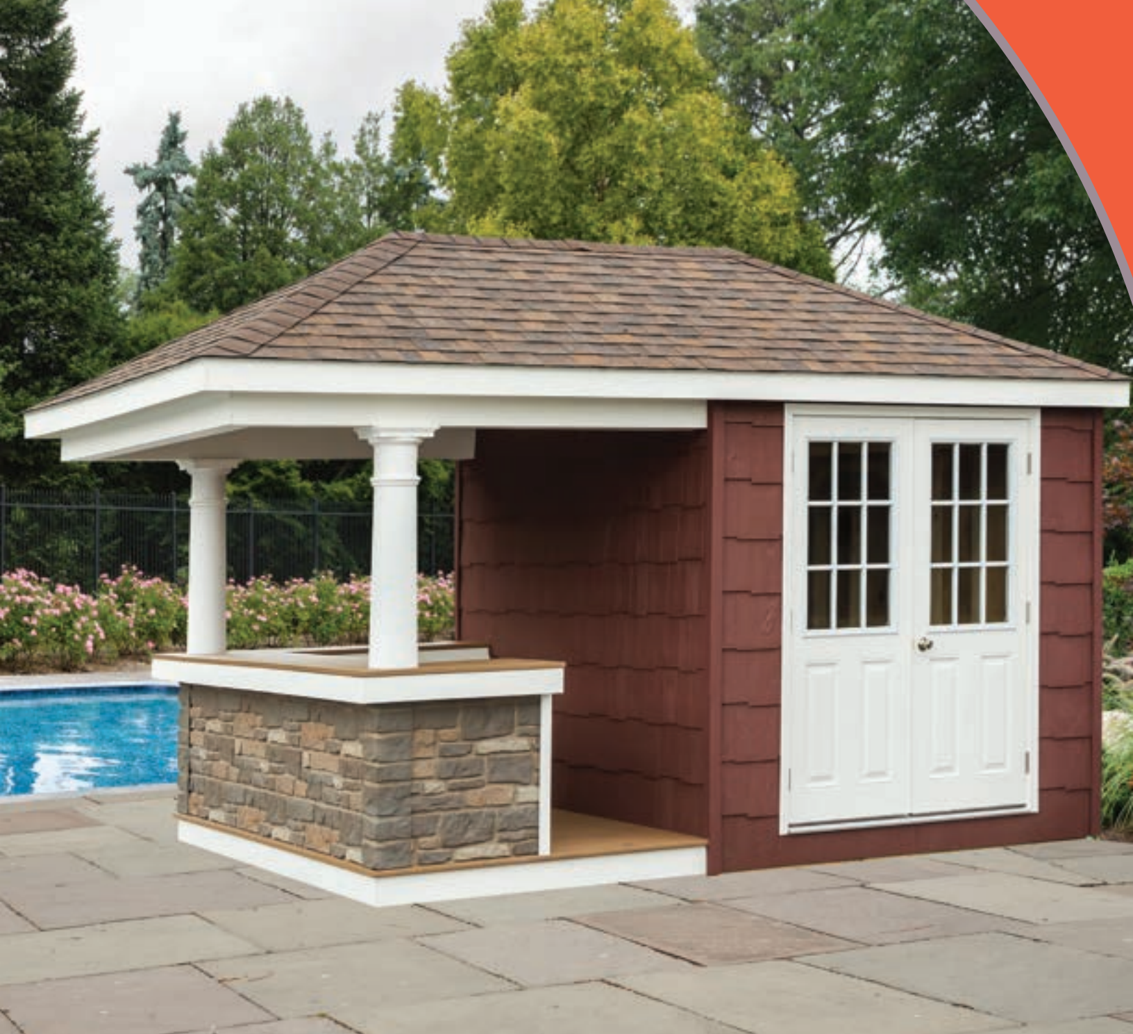
Shown with rustic redwood shingles and teakwood decking
