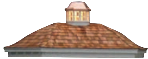
Cedar Shake Roof
